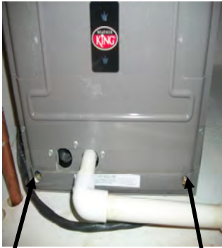
Access to air filter (Condos)
